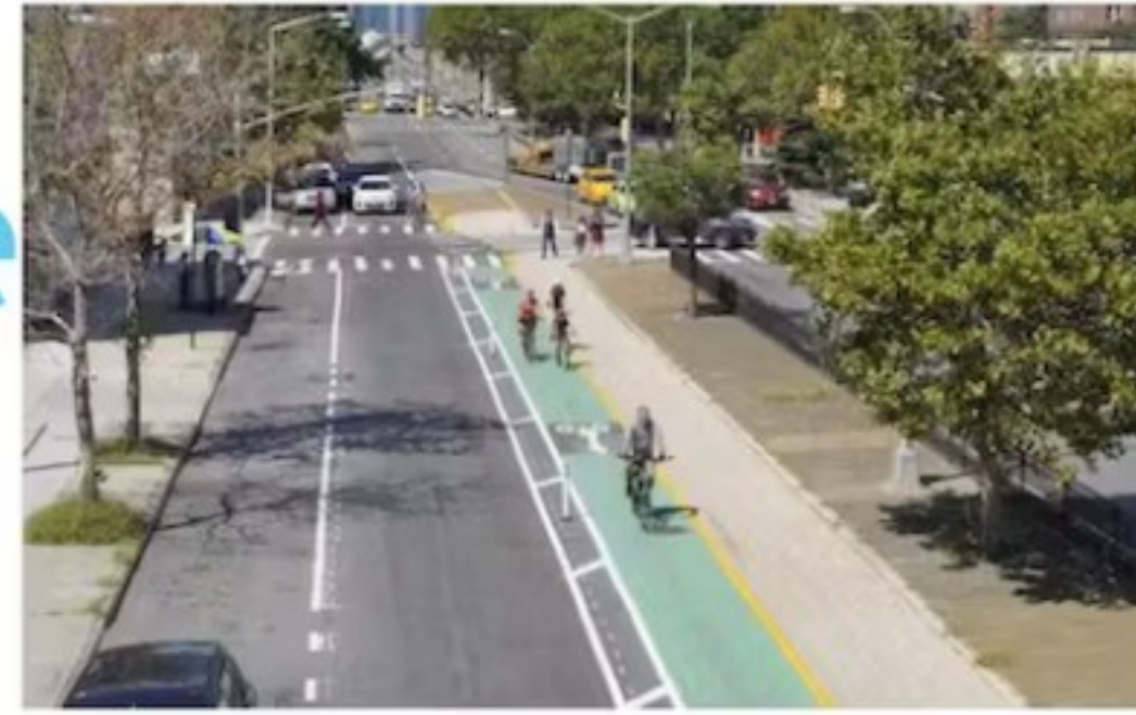
4. Striped bike lanes along vehicular lanes with a separate sidewalk for pedestrians
