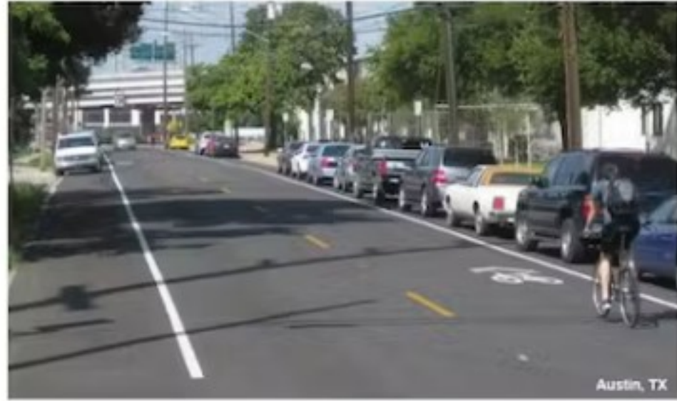
1. Sharrow – Lanes shared by vehicular traffic and bikes with separate sidewalks for pedestrians
